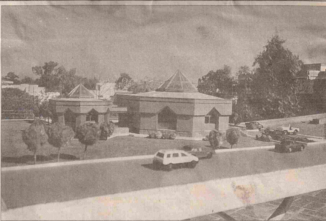
MULTAN: The model of 'Police service counter' building to be built at the Qasim Bagh Fort — Dawn
